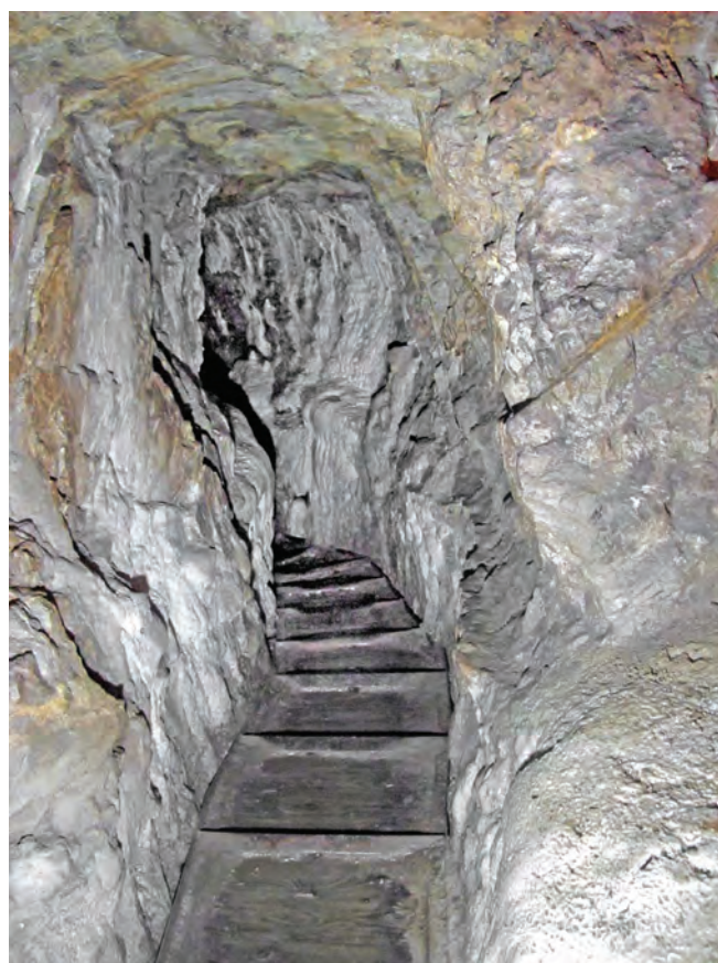
The narrow twisting passage within the mediaeval drainage adit at Kutna Hora
